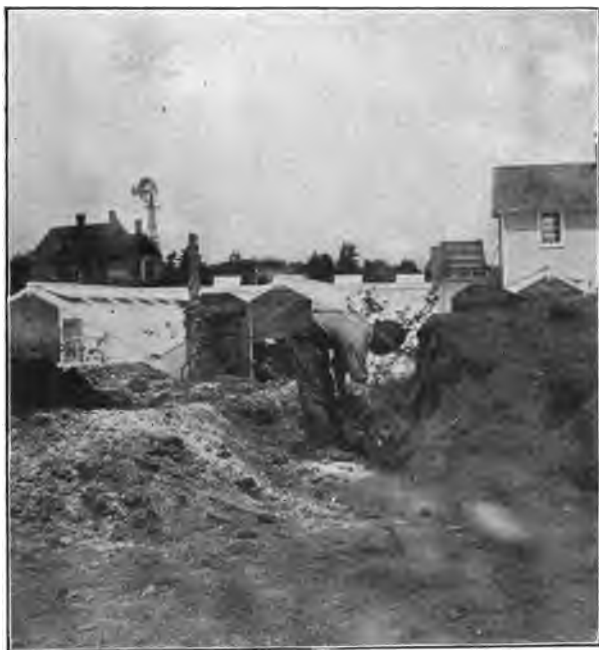
5.— Mixing soil. Breaking and pulverizing the sod preparatory to putting it down with layers of manure.
